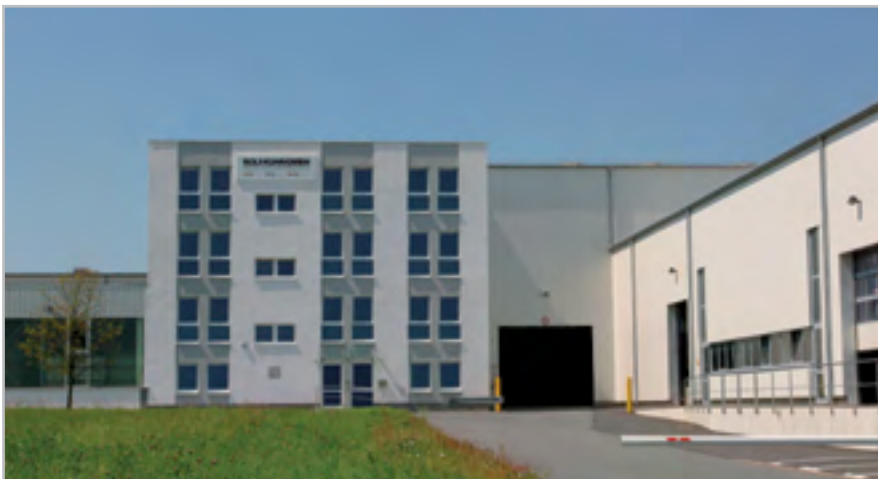
The factory of the Rolf Kuhn GmbH in Erdtebrück.
